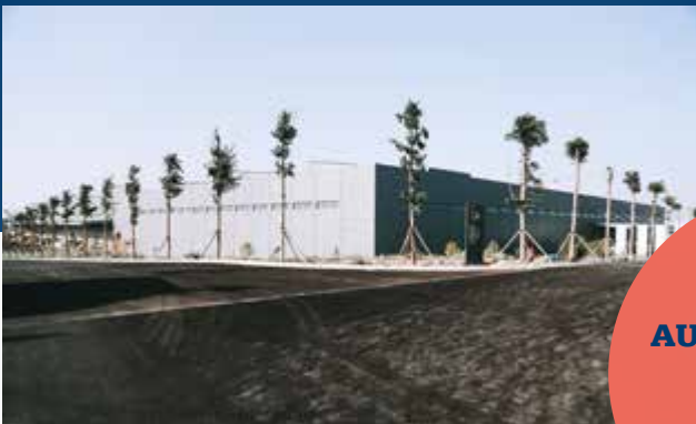
EXTERIOR VIEW of the Saurer production site in China
